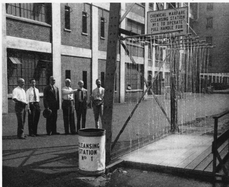
Left to right, Walter Racicot, Milt Burrall, Dr. Smith, Burt Hine — all of Scovill — Dr. O'Brien of the State Defense Council, and Wallace Bergstrom of the Scovill A.R.P. organization look at the Chemical Warfare Cleansing Station just outside the Grinding Room in Building 49. This is one of several similar stations for use of those who might be caught in an enemy gas attack.
