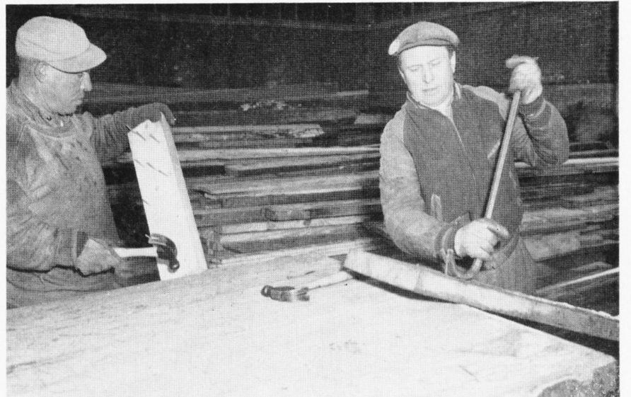
On nearly every job there is lumber left over when scaffolds are removed, when forms for concrete have done their work. A couple of fellows from the Yard Department are shown removing nails from used lumber. They're Antonio Insogna — four of his sons are in the Army — and Joe Nebiolo. The lumber they are reclaiming will be used over and over again, as long as it is safe and serviceable. How many of these economies can you use at home?
